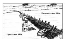
Fig.2. Single line simple weir.
